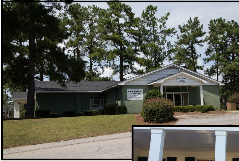
Repairs at Livingston House & the Canteen
