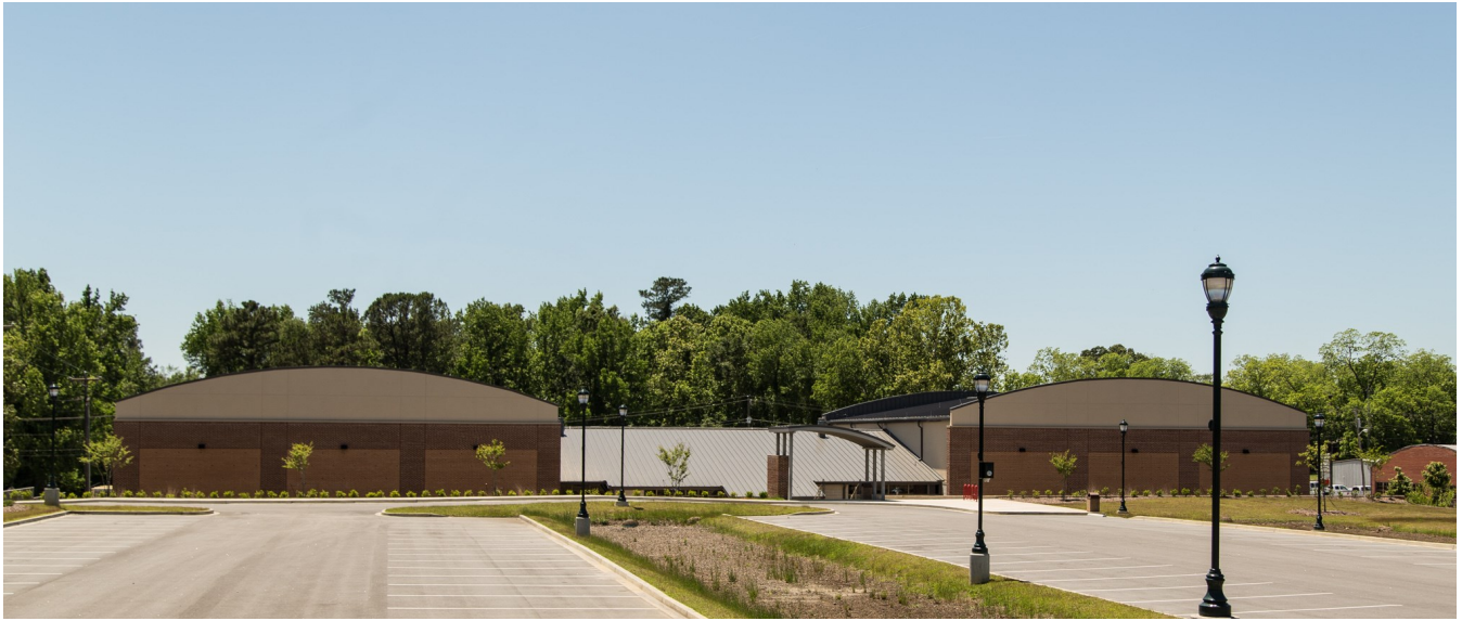
Construction of New City Gym
