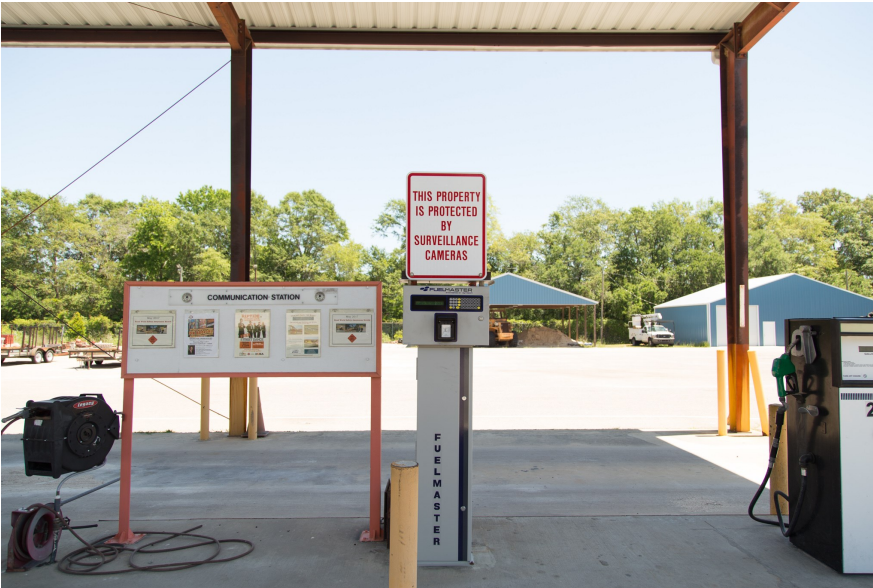
New Fuel Station
