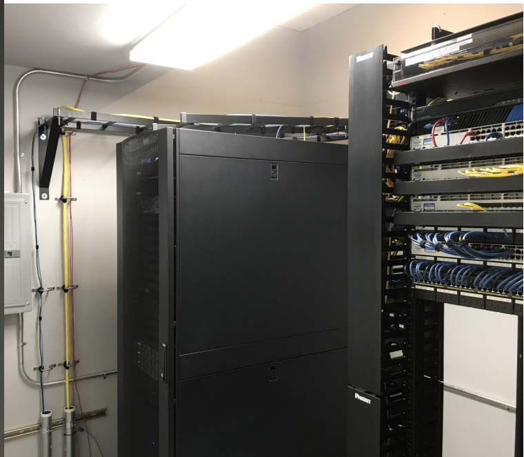
Repairs & Upgrades to IT Server Room
